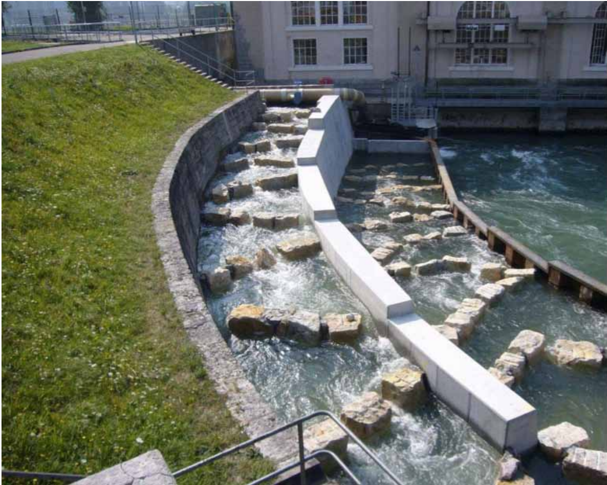
Fish passage at the Wyhlen hydroelectric power plant in Baden-Württemberg
