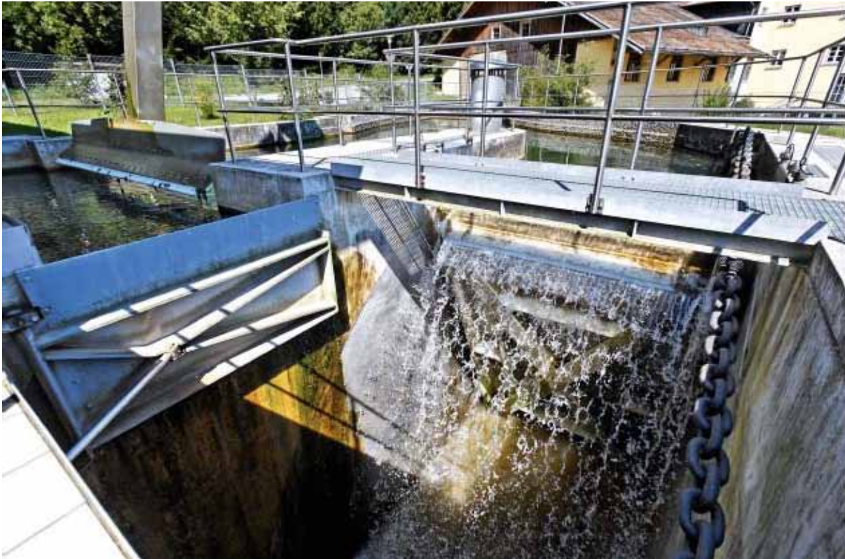
A hydroelectric power system in the district of Traunstein, Bavaria
