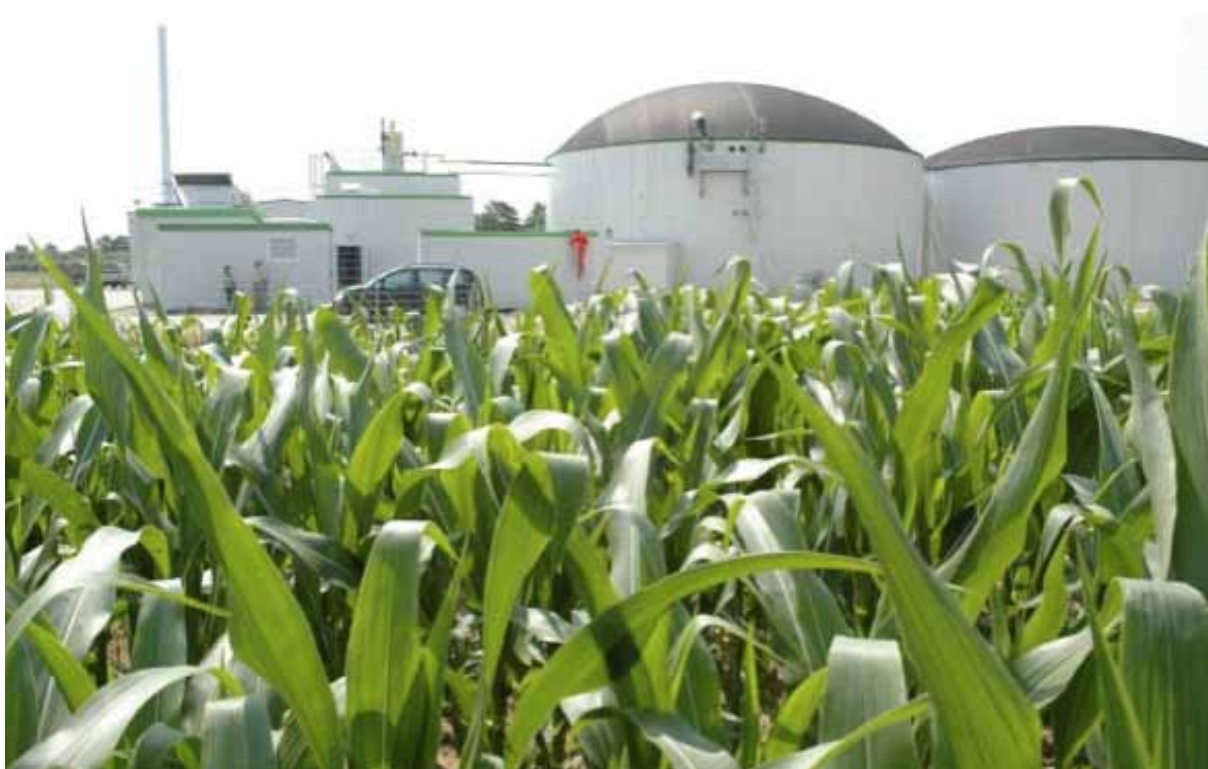
Modern biogas system
